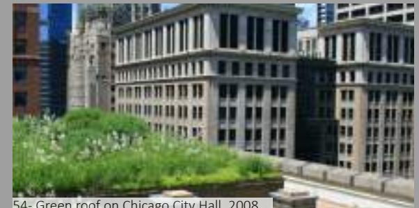
54- Green roof on Chicago City Hall, 2008.
